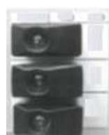
Figure 2 – Voltage presence indicators
